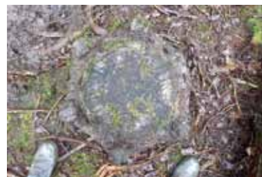
写真-49 笠上部直径510mm 厚さ175mm
